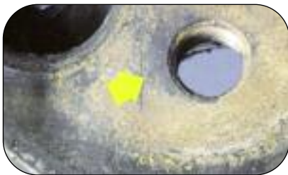
Figure 2 - Damaged Core Refund Bottom deck crack
